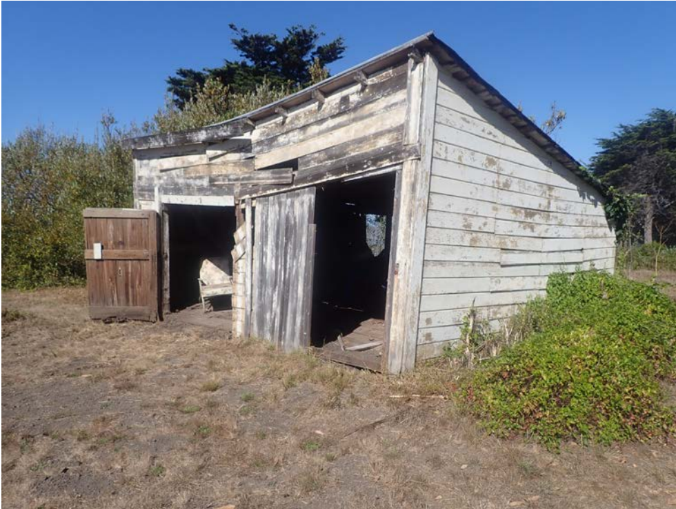
Figure 7. Carriage house / garage post modification.
