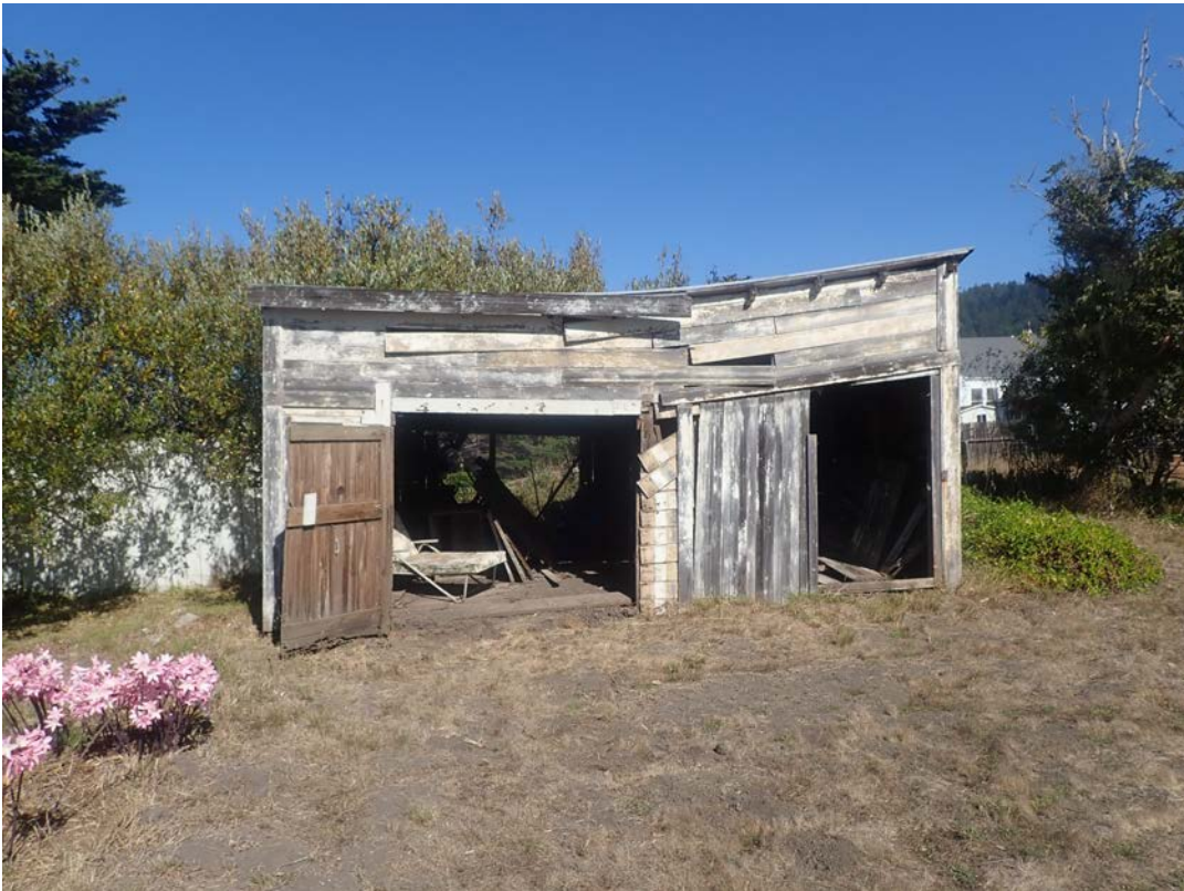
Figure 6. Carriage house / garage post modification.
