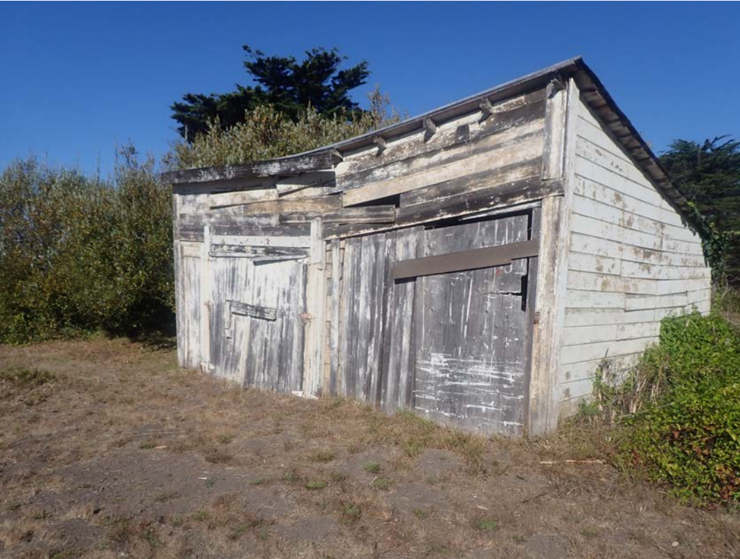
Figure 3. Carriage house / garage exterior before modification.
