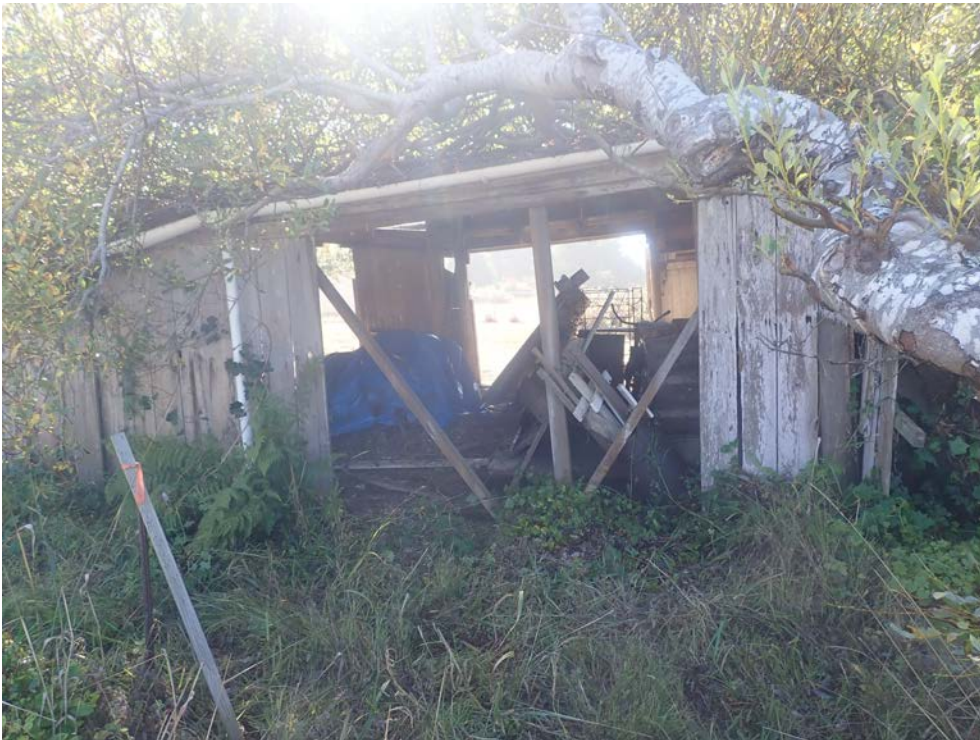
Figure 8. Carriage house / garage post modification from the north looking south.
