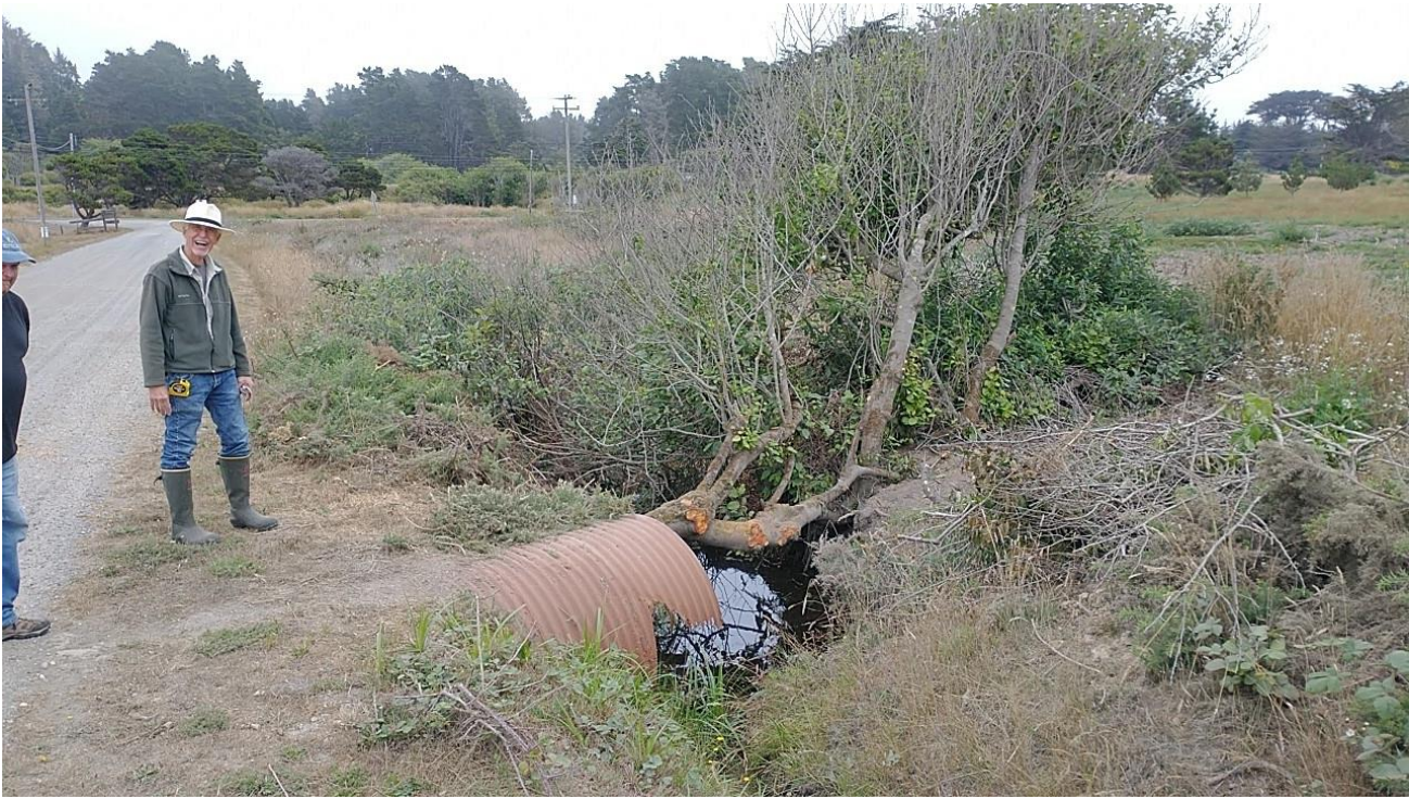
Photo 4. Culvert inlet standing on the west side
