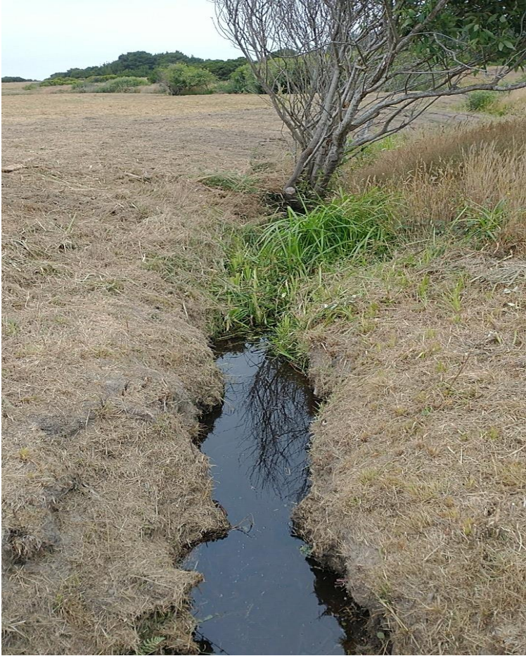
Photo 2. Channel immediately downstream of culvert outlet
