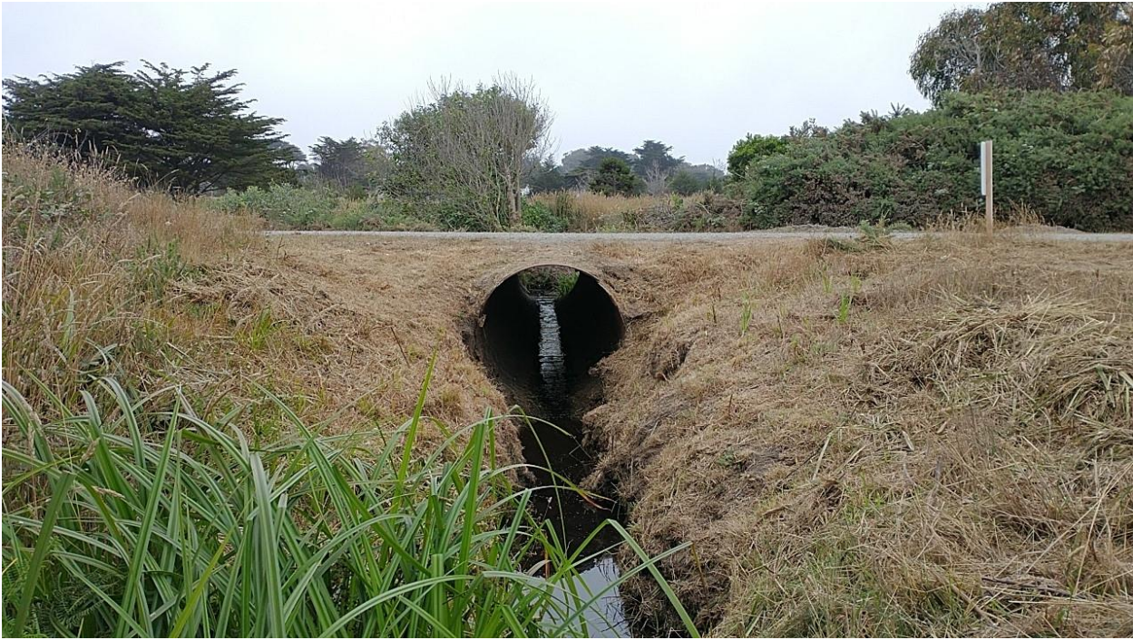
Photo 1. Downstream of culvert facing upstream
