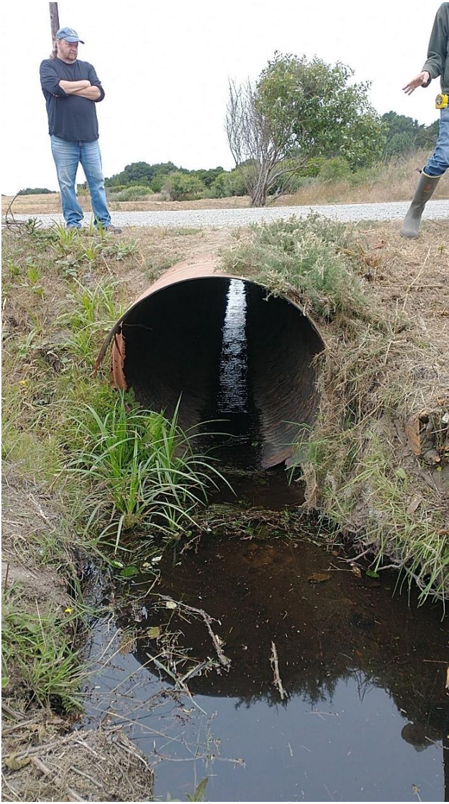
Photo 3. Culvert inlet facing downstream
