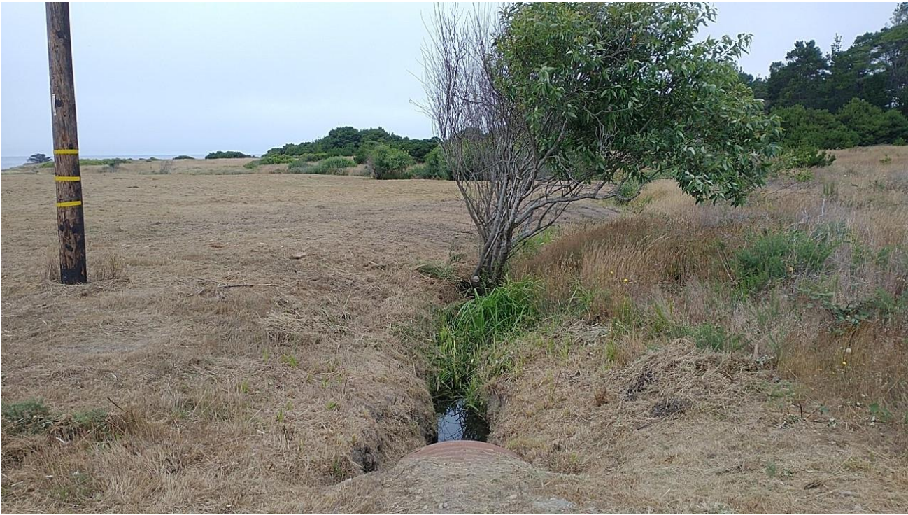
Photo 6. Downstream channel below culvert outlet
