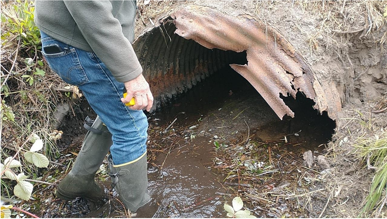
Photo 5. Caspar Road culvert outlet facing upstream
