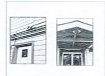
EXISTING EXTERIOR LIGHTS
