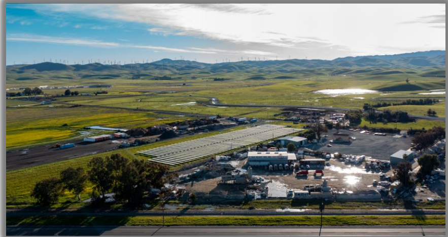
Byron Hot Springs Road Solar Contra Costa County, CA
