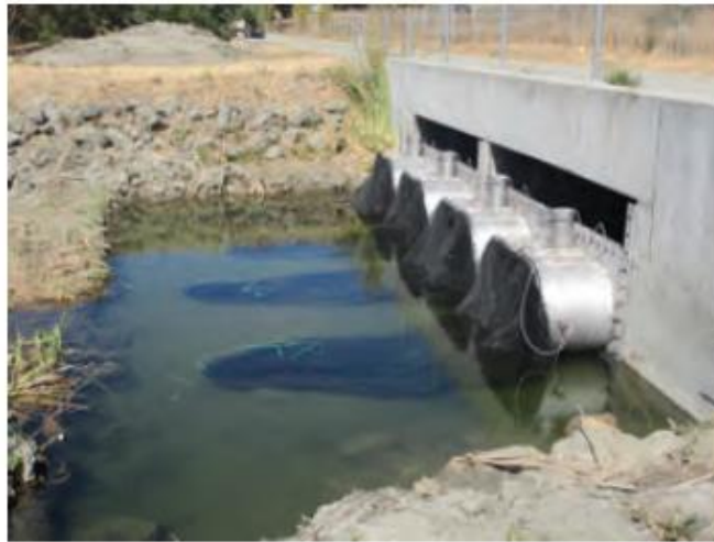
Representative Image 4. Example of End-of-Pipe Netting System
