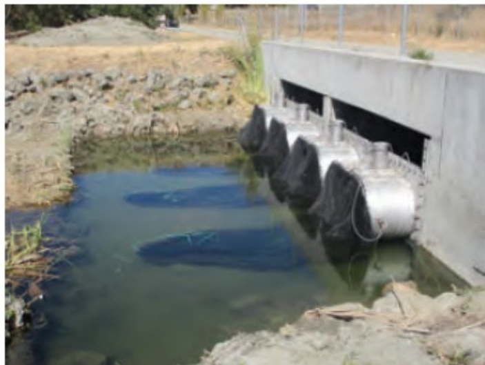
Figure 5. Example of End-of-Pipe Netting System
