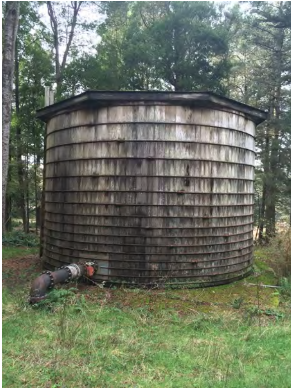
Existing Redwood Tank
