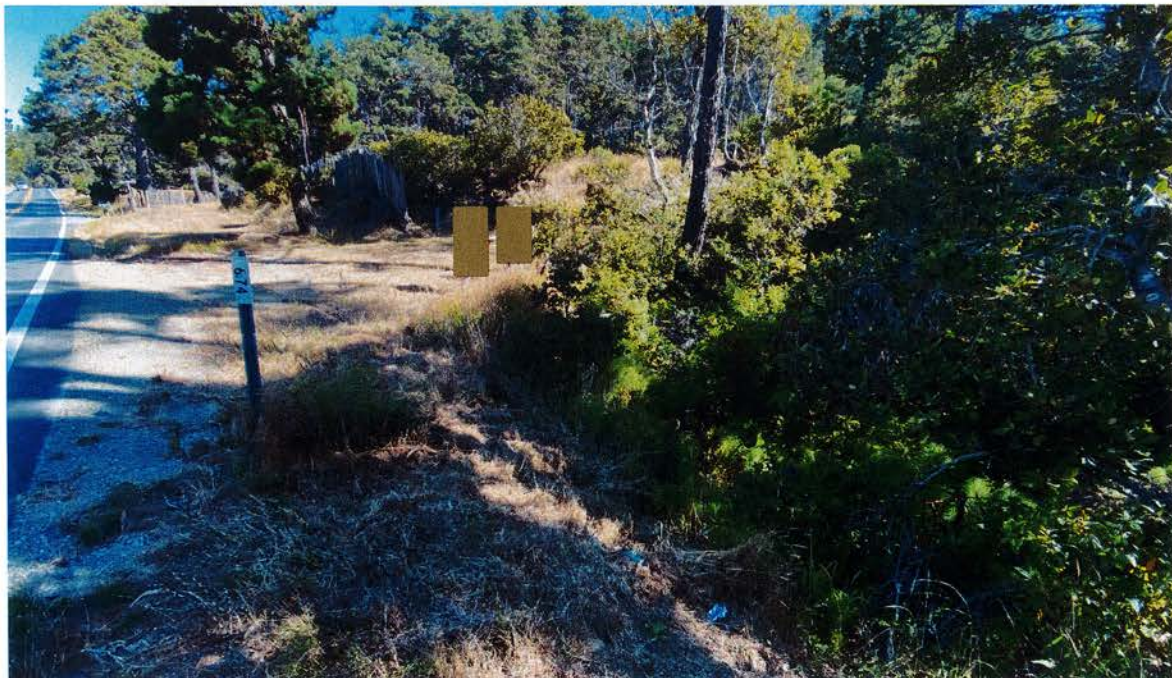
Photo 6. View of culvert at PM 6.74, looking north. Riparian area and future Reveg Area 4. Date of photo: August 18, 2022.
