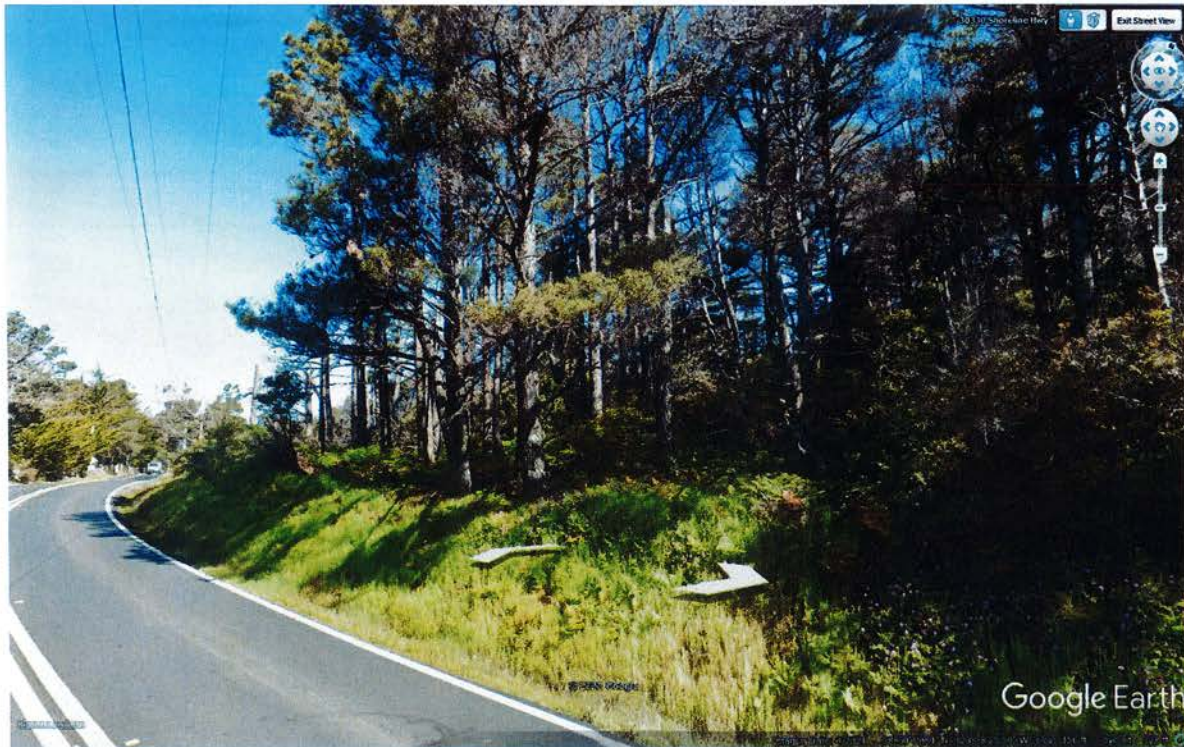
Photo 7. View of upland proposed road cut at approximate PM 9.44, looking northeast. Bishop pine forest and future Reveg Area 6. Date of Google Earth Street View Image: April 2021.
