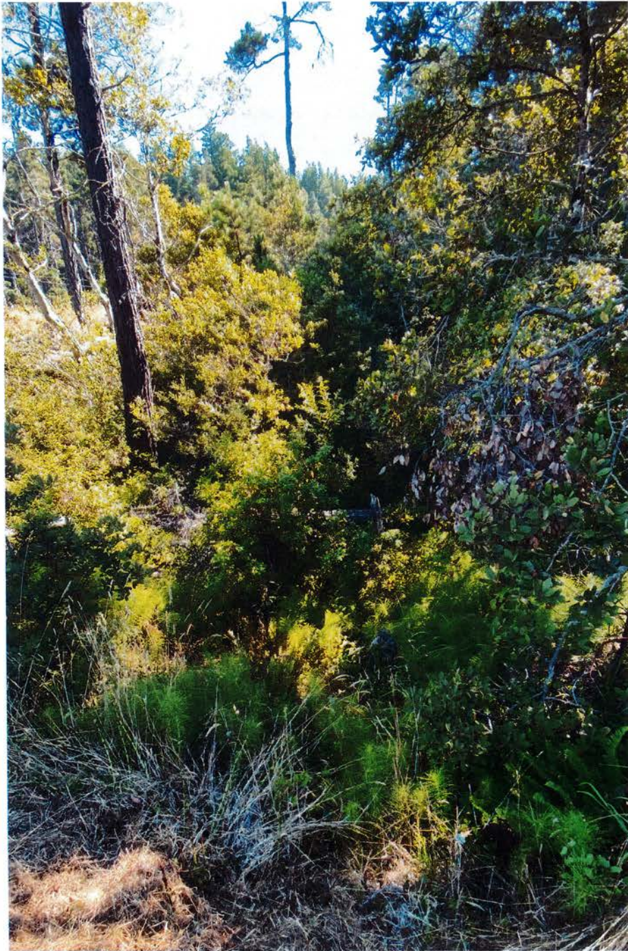
Photo 6. View of culvert at PM 6.74, looking east. Riparian area and future Reveg Area 4. Date of photo: August 18, 2022.
