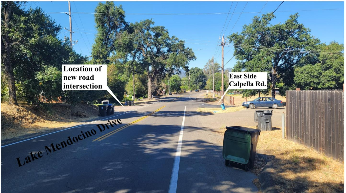
Figure 2. Alignment Option B. Lake Mendocino Drive looking West. The potential new road intersection B, as labeled on map, is proposed to be on the South side of the road.
