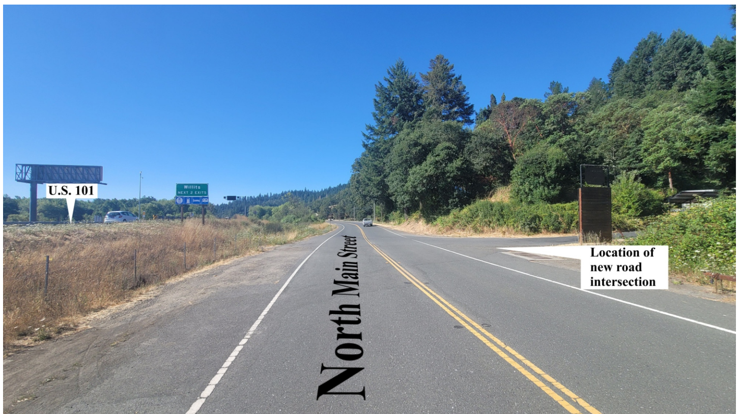
Figure 2. North Main Street looking south. The proposed new road location is to be located on the West side of the road.
