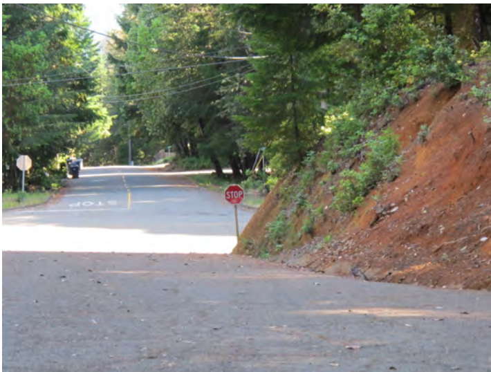
Photo Location 12: Looking south and west; road cut consisting of intensely weathered rock/residual soil.
