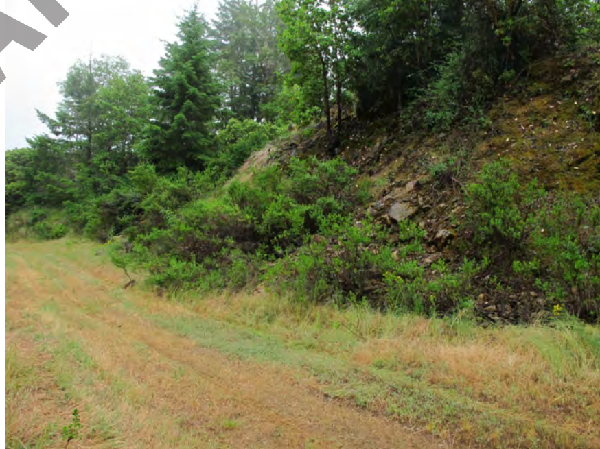
Photo Location 6: Looking southeast, angular bedrock exposed in road cut, drainage ditch on inboard side of road uphill of waterbar.
