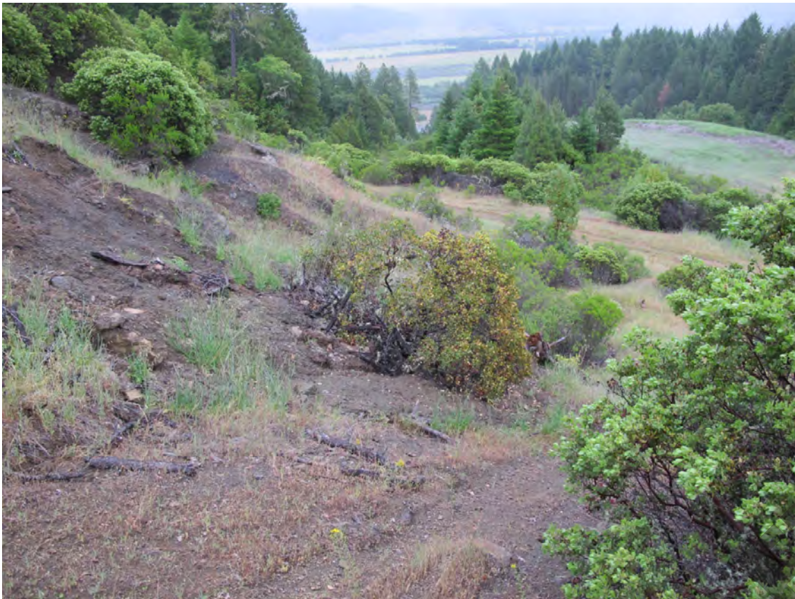
Photo Location 3: Looking south; fresh slide scarps, location 10 in the upper right corner of lower picture.
