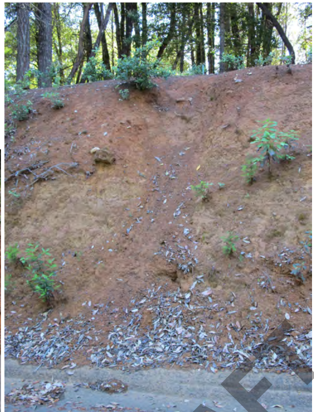
Photo Location 12: Looking south and west; road cut consisting of intensely weathered rock/residual soil.
