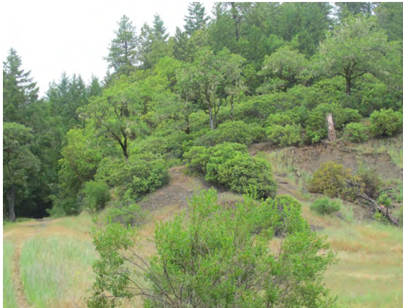
Photo Location 2: Looking north towards location 3; recent slide activity and southeast end of existing FirCo haul road crossing steep terrain.
