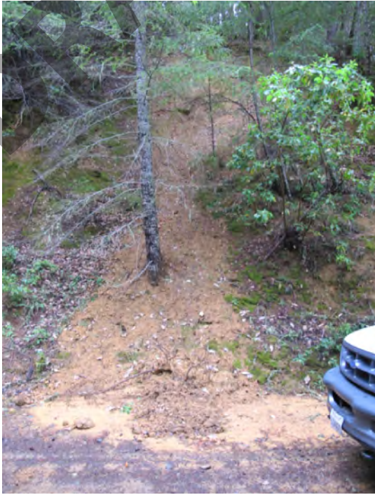
Photo Location 3a: Photos of debris flow along road cut.
