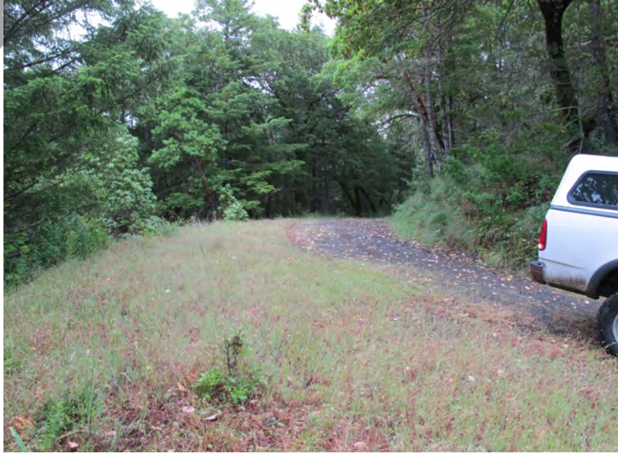
Photo Location 7: Looking east. Bedrock exposed in road surface.
