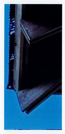
10-year-old steel roof (yes, that is holes in the steel)
