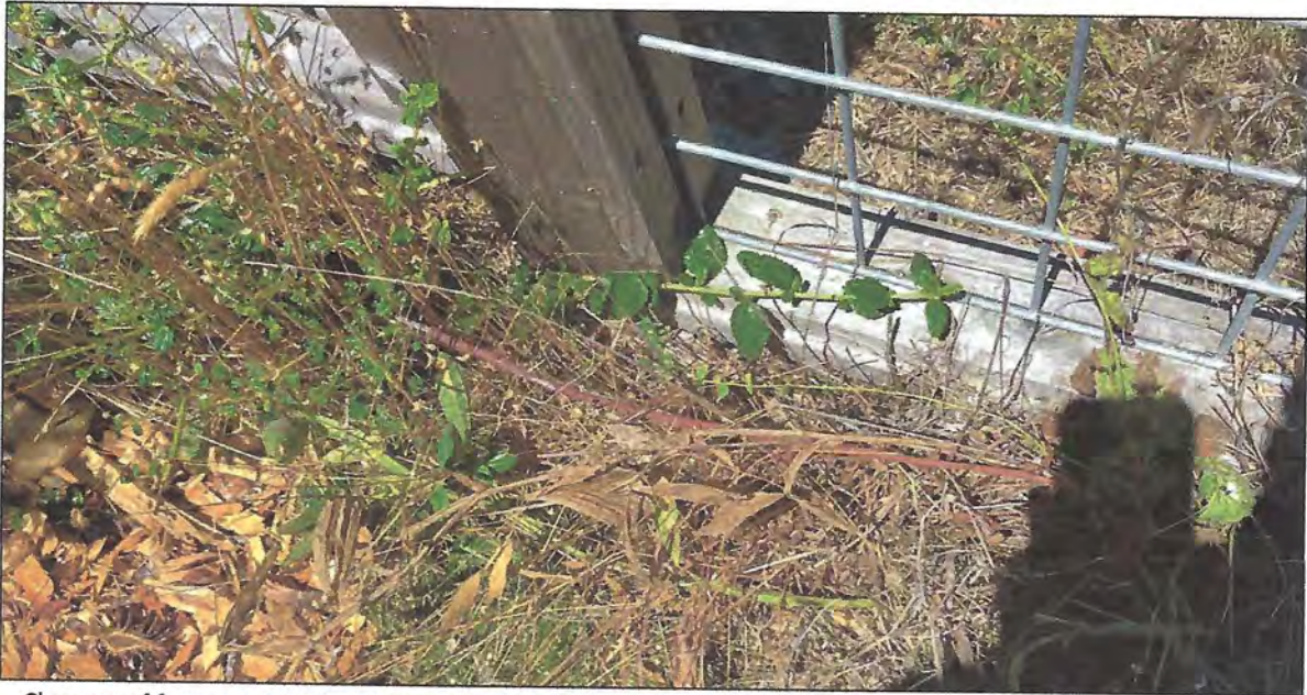
Close-up of fence post contact with ground; note vegetation growing up to and cover surface expression of fence post footing; note no side cast soil, sediment migration, or erosion
