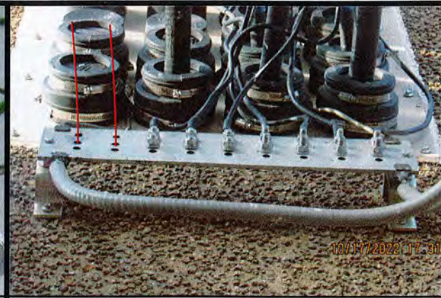
EXISTING OUTSIDE SHELTER
