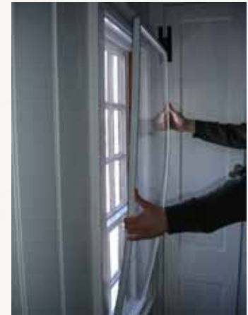
Interior storm panel.
