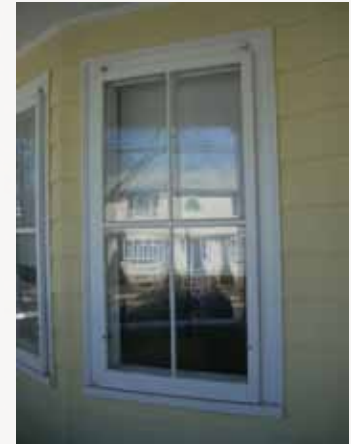
A traditional wood storm window fastened by hangers at the top. This storm window is also secured by four screws along the perimeter.
