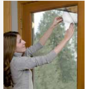
Homeowner installation of low-e interior surface film.
