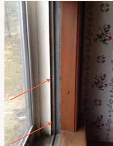
The red arrows indicate metal weather stripping that fits into a routed channel along the sides and bottom of the sash.
