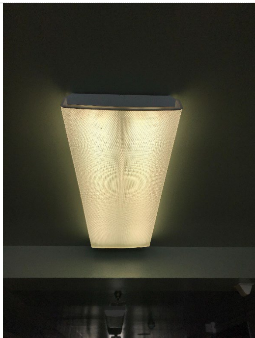
Photo #15: Light fixture – Lithonia Lighting Model: LB 32 MVOLT ¼ MVIS
