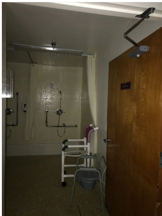
Photo #9: Shower room - ceramic tile floor, baseboard and walls
