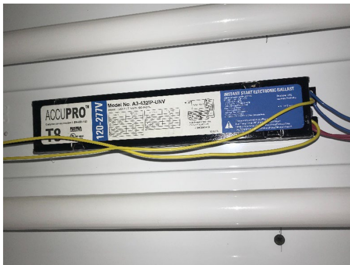
Photo #16: Ballast Model No. A3-432IP-UNV Type 1 Outdoor, No PCB's
