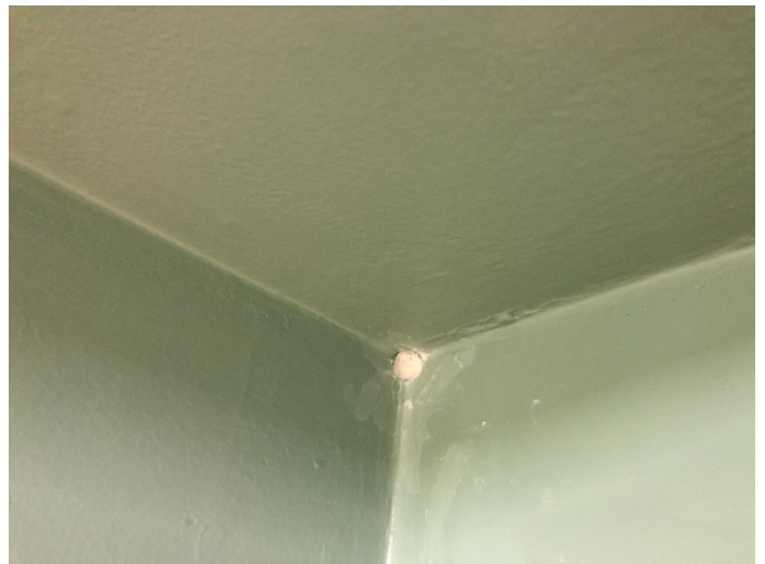
Photo #4: Interior drywall with joint compound sampled (63797-101-01 to 03)
