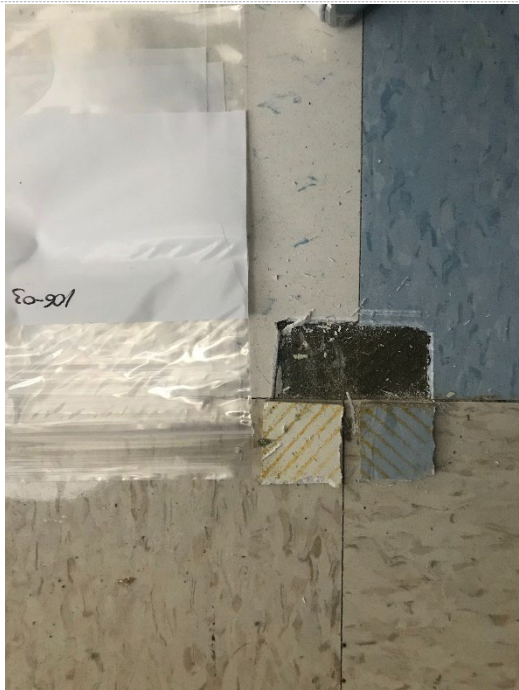
Photo #5: Black and yellow mastic; Blue, off white and beige 12"x12" vinyl floor tile
