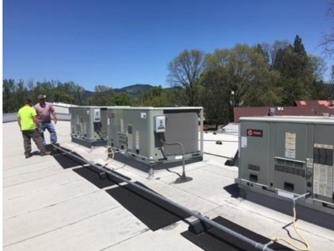
Figure 12. New roof and new HVAC units at Exhibit Building Roof
