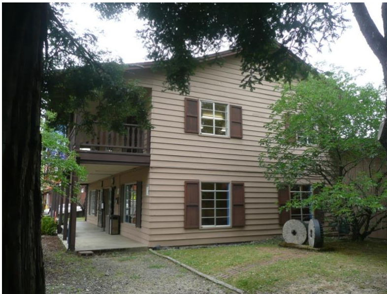
Figure 1. Administration Building East Elevation
