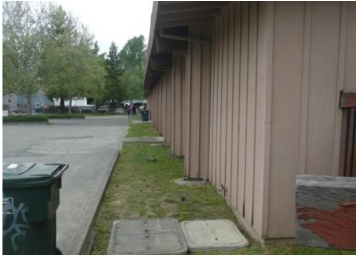
Figure 6. Drainage at West Elevation
