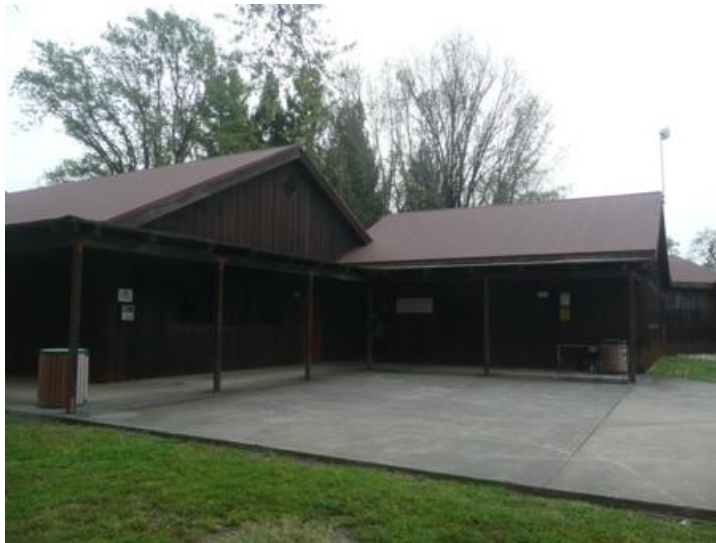
Figure 10. North Elevation, Rear entry to Classroom Building
