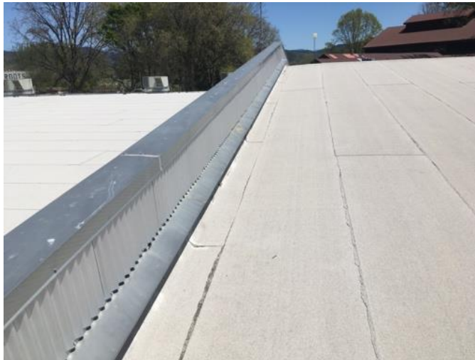
Figure 13. Parapet at seismic joint between Exhibit Building and Collections Storage Building
