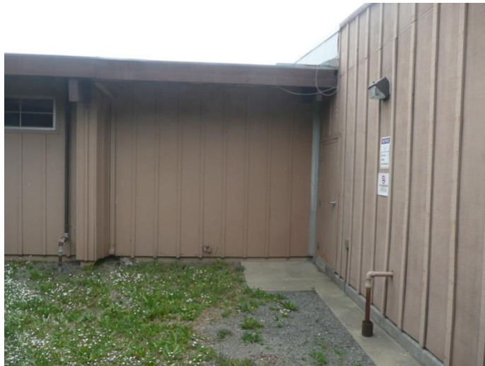
Figure 19. Plywood with batten siding at Exhibit and Collection Storage Buildings
