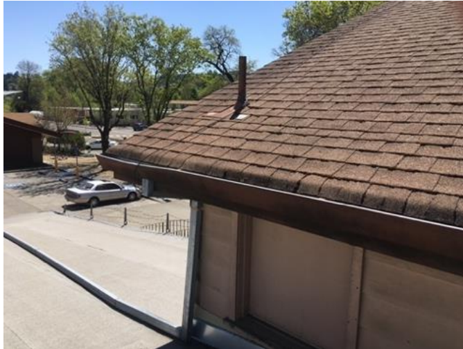
Figure 11. Composition shingle roof at Administration Building
