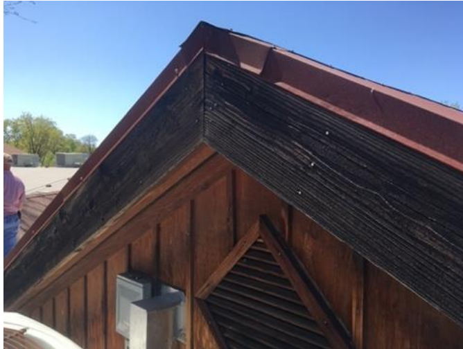
Figure 20. Untreated and weathered redwood siding and trim at Classroom Building
