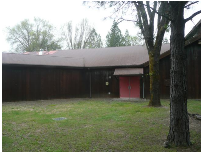
Figure 33. Potential entry to Classroom Building from south side of building.
