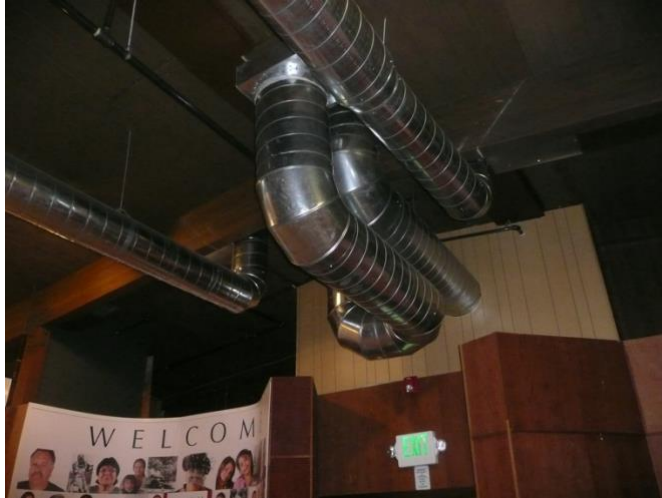
Figure 23. New ductwork at Exhibit Building
