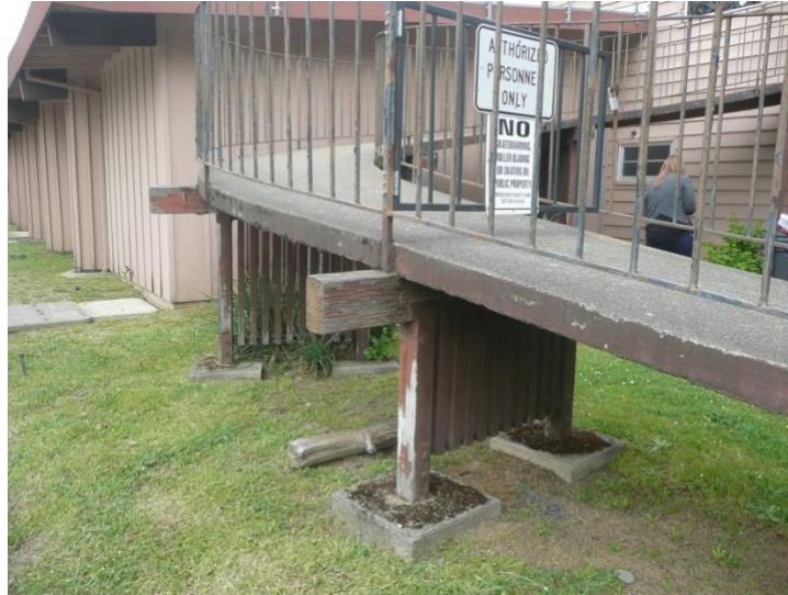
Figure 5. Curved Ramp to Second Floor
