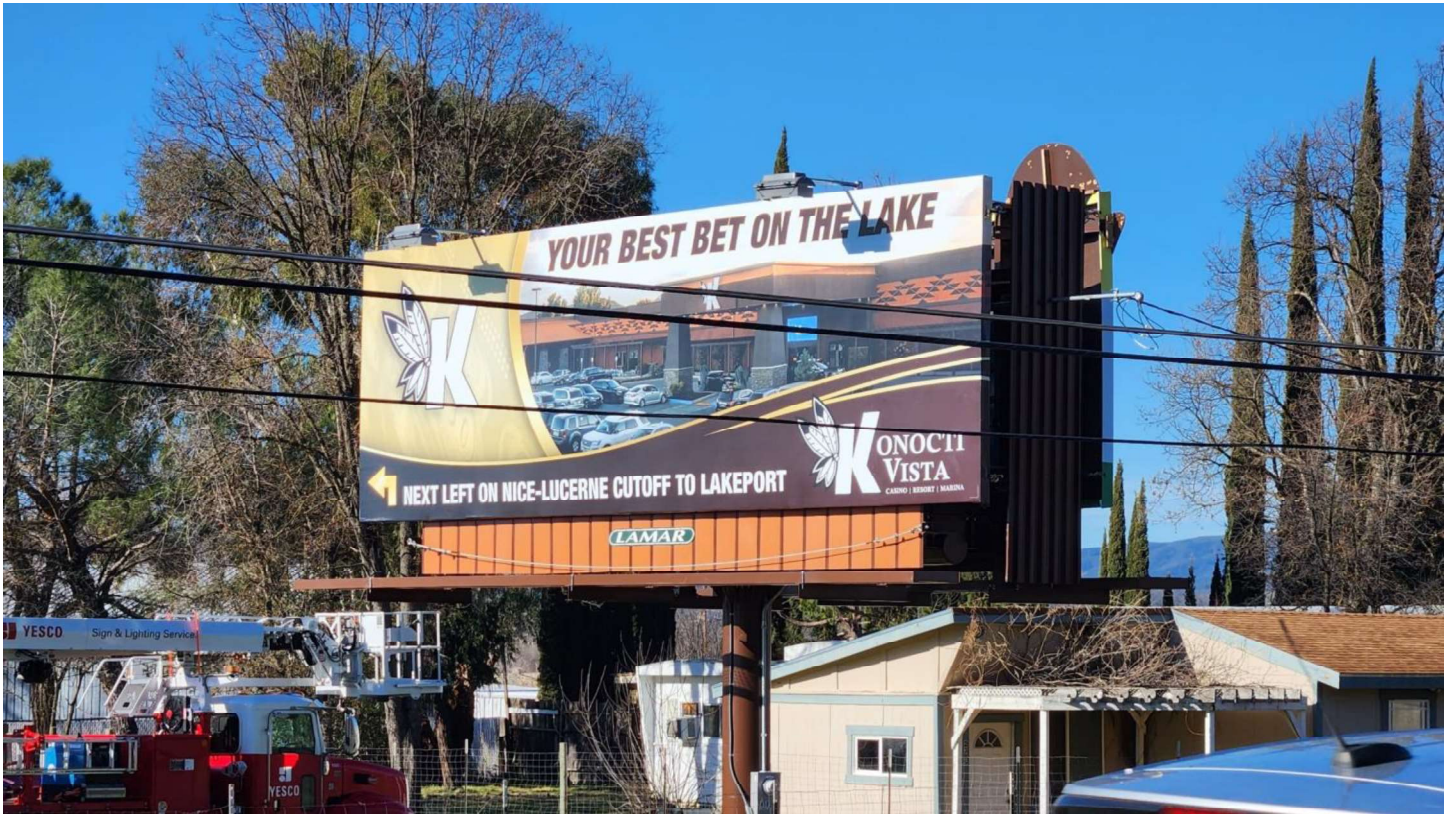
Example of sign fitted with top-mounted luminaires and accessory light shields
