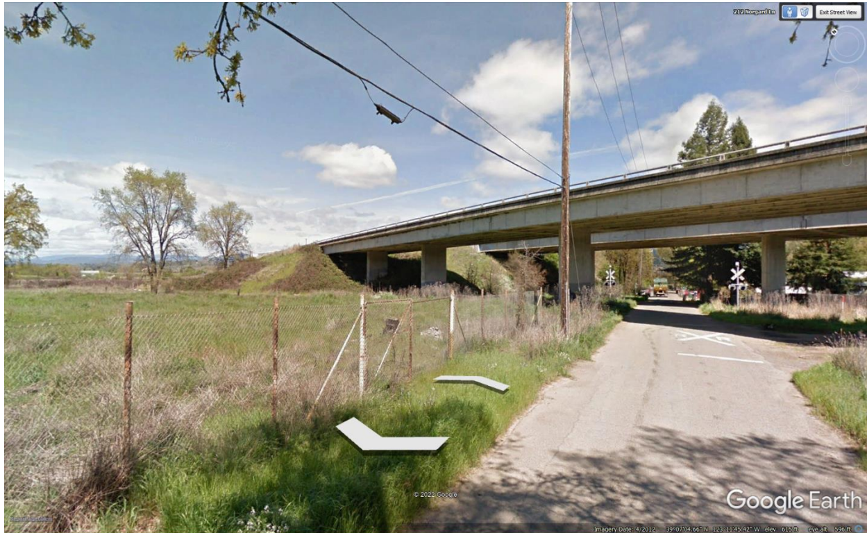
Figure 4 - View of the overpass from Norgard Ln. (Provided by Staff)
