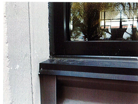
NEW ALUMINUM WINDOW FRAMES USED ON GYMNASIUM TO MATCH PHASE 1 - DARK BRONZE
