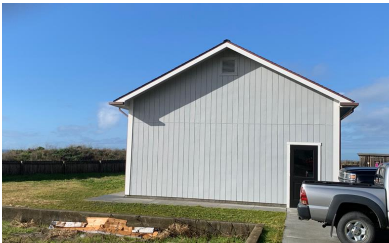
MCCSD Building with Plywood Siding & Aluminum Windows
