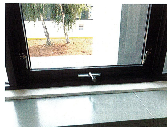
NEW ALUMINUM WINDOW FRAMES USED ON GYMNASIUM TO MATCH PHASE 1 - DARK BRONZE
