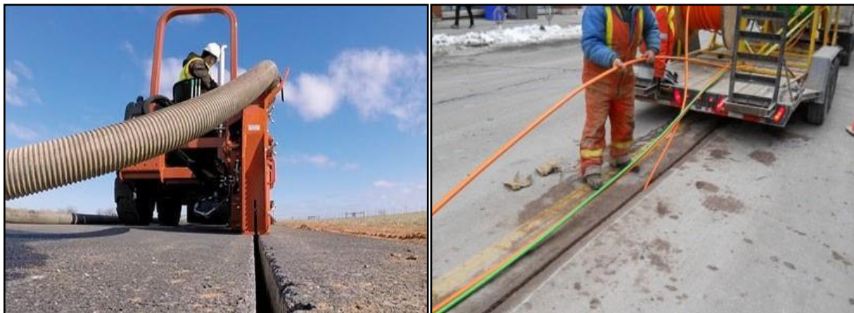
Figure 1. Micro-trenching
