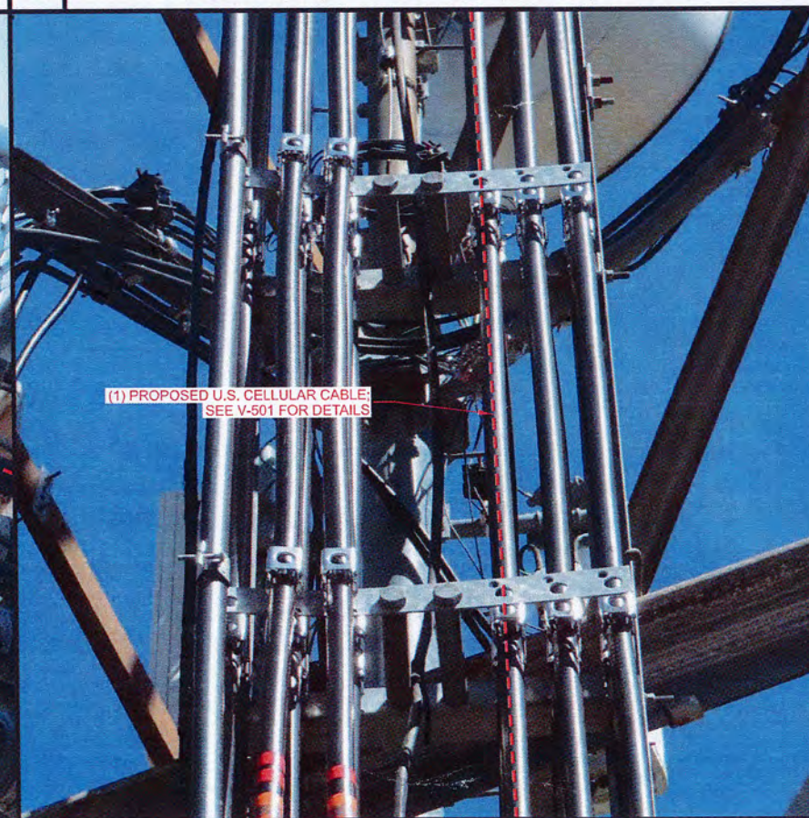
E CABLE ROUTING UP TOWER FACE
