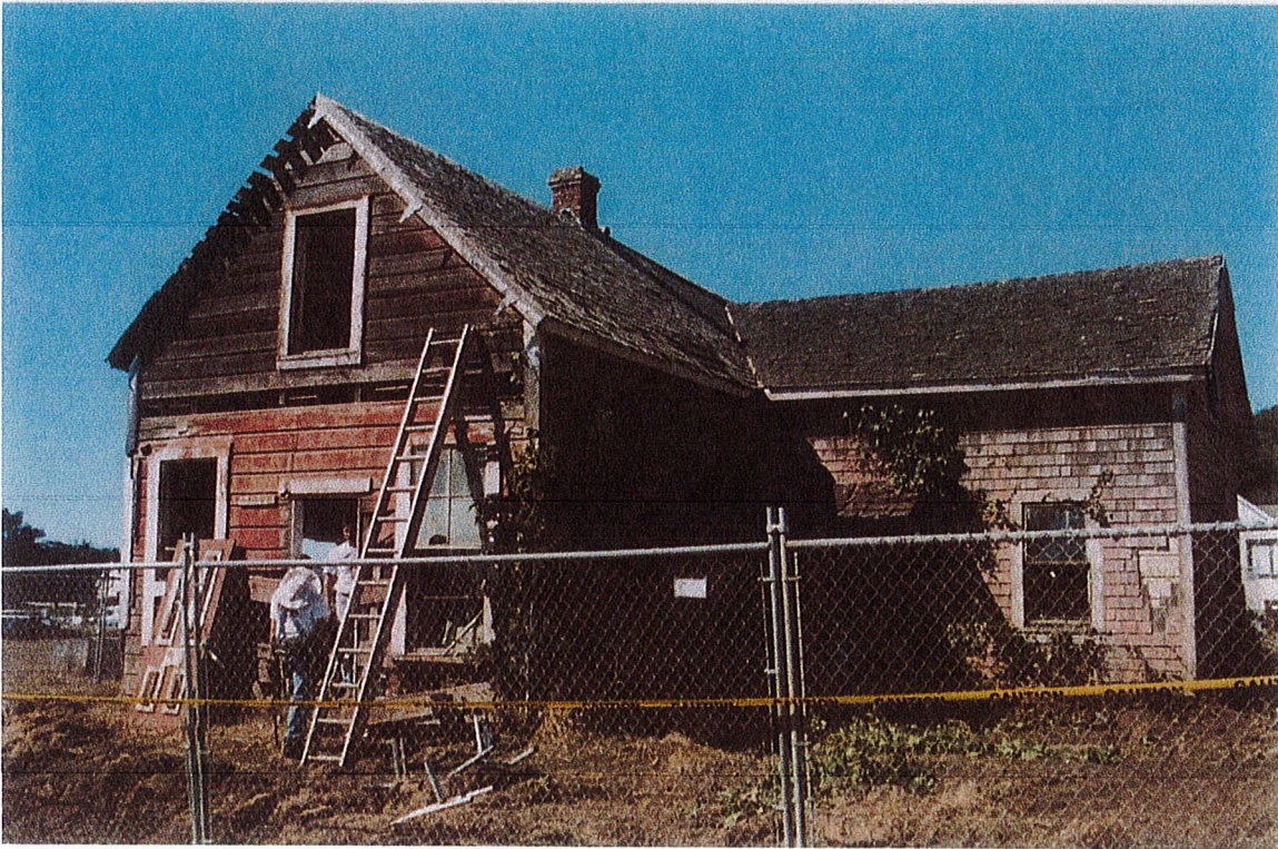
The 'Rego' house beginning the demolition
