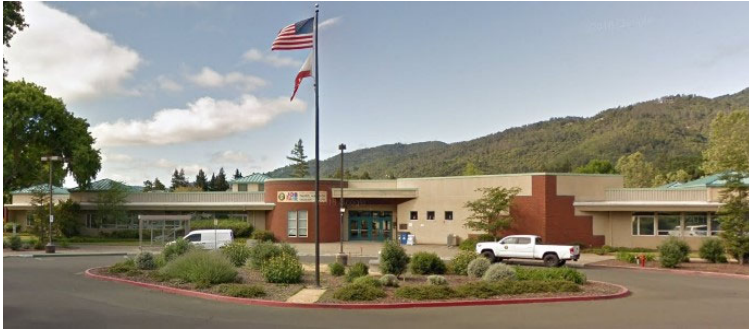
Mendocino County Administration Center, Ukiah, CA
