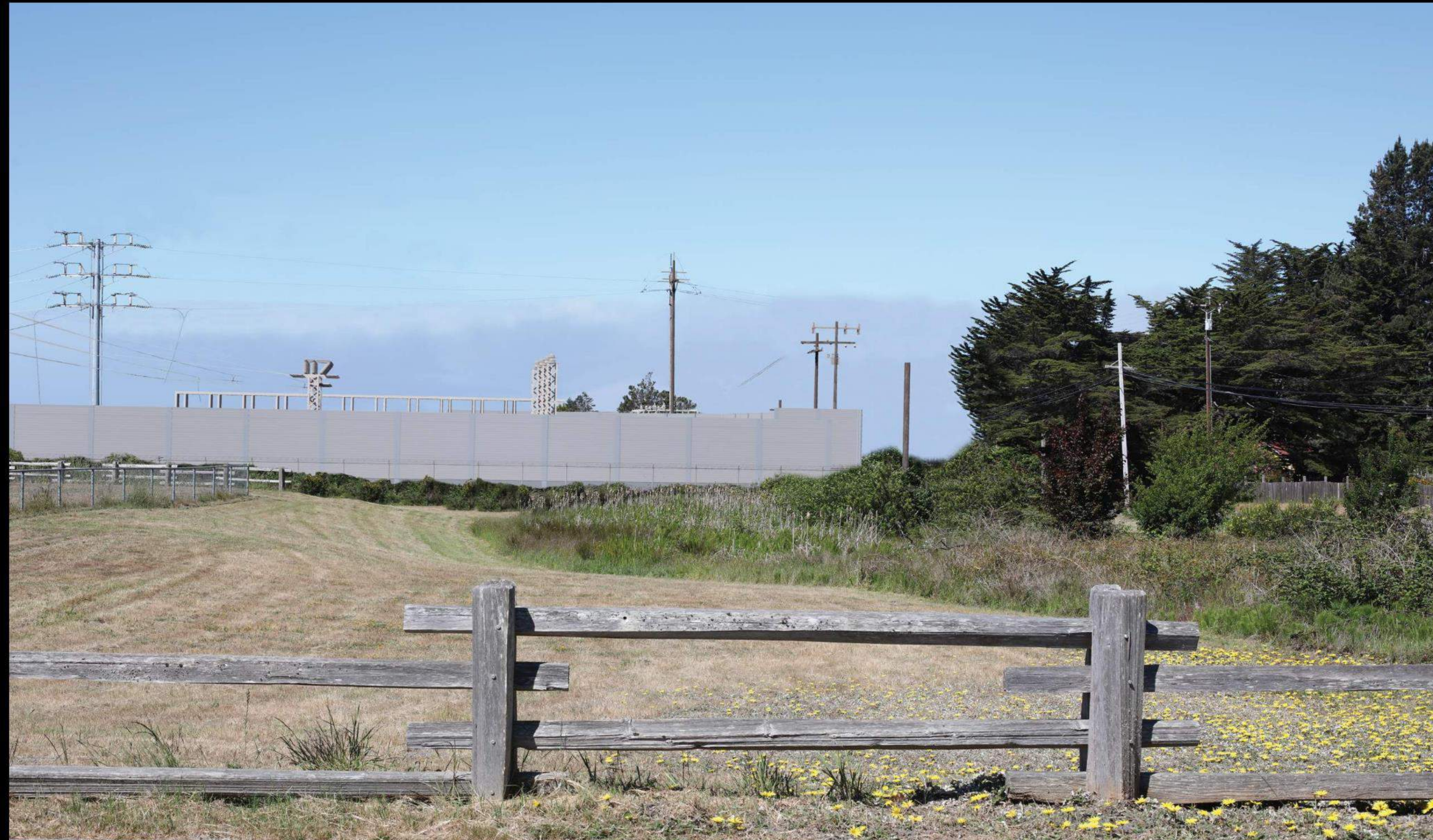
EXISTING WALL / VEGETATION REMOVED
