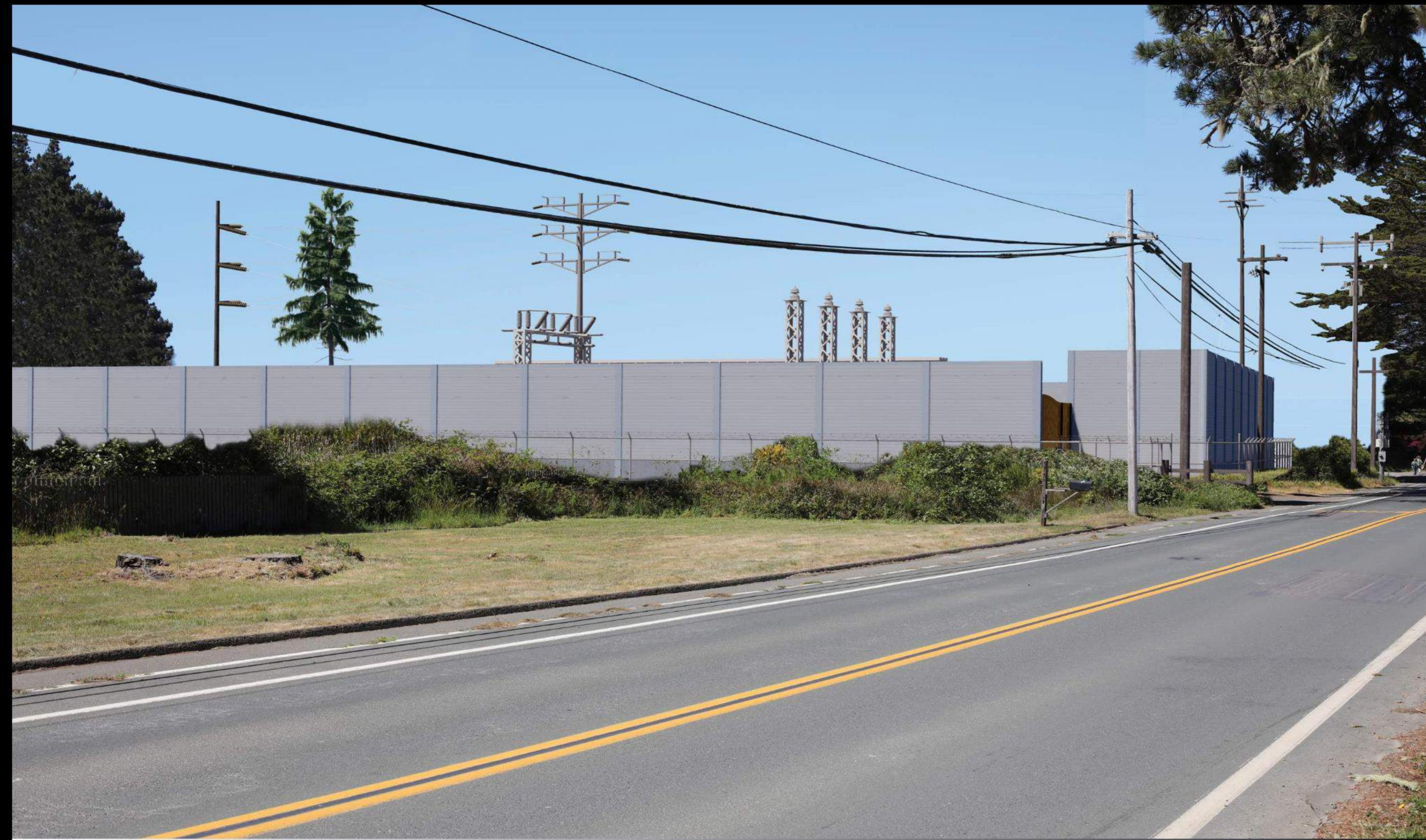
EXISTING WALL / VEGETATION REMOVED
