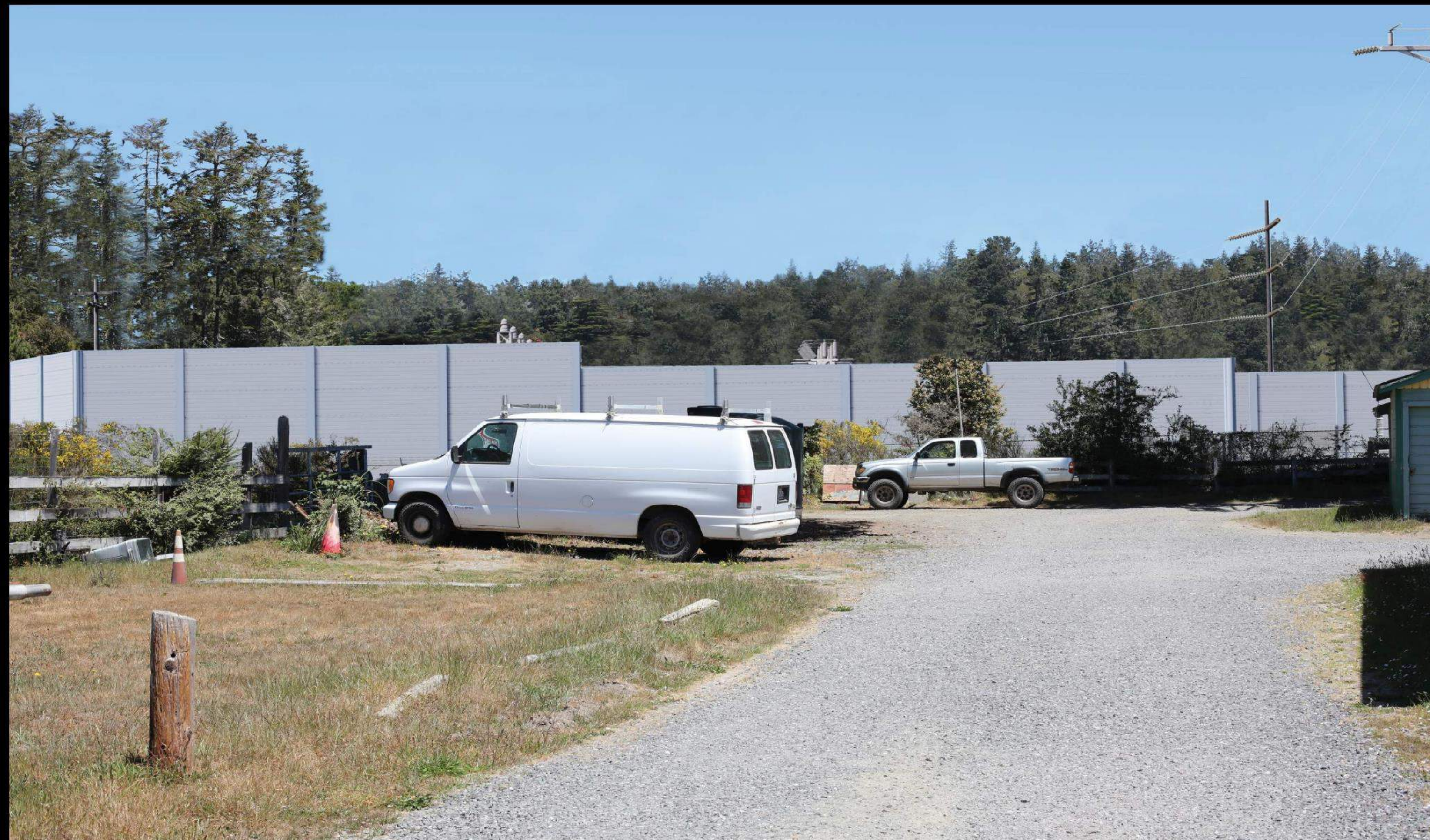
EXISTING WALL / VEGETATION REMOVED
