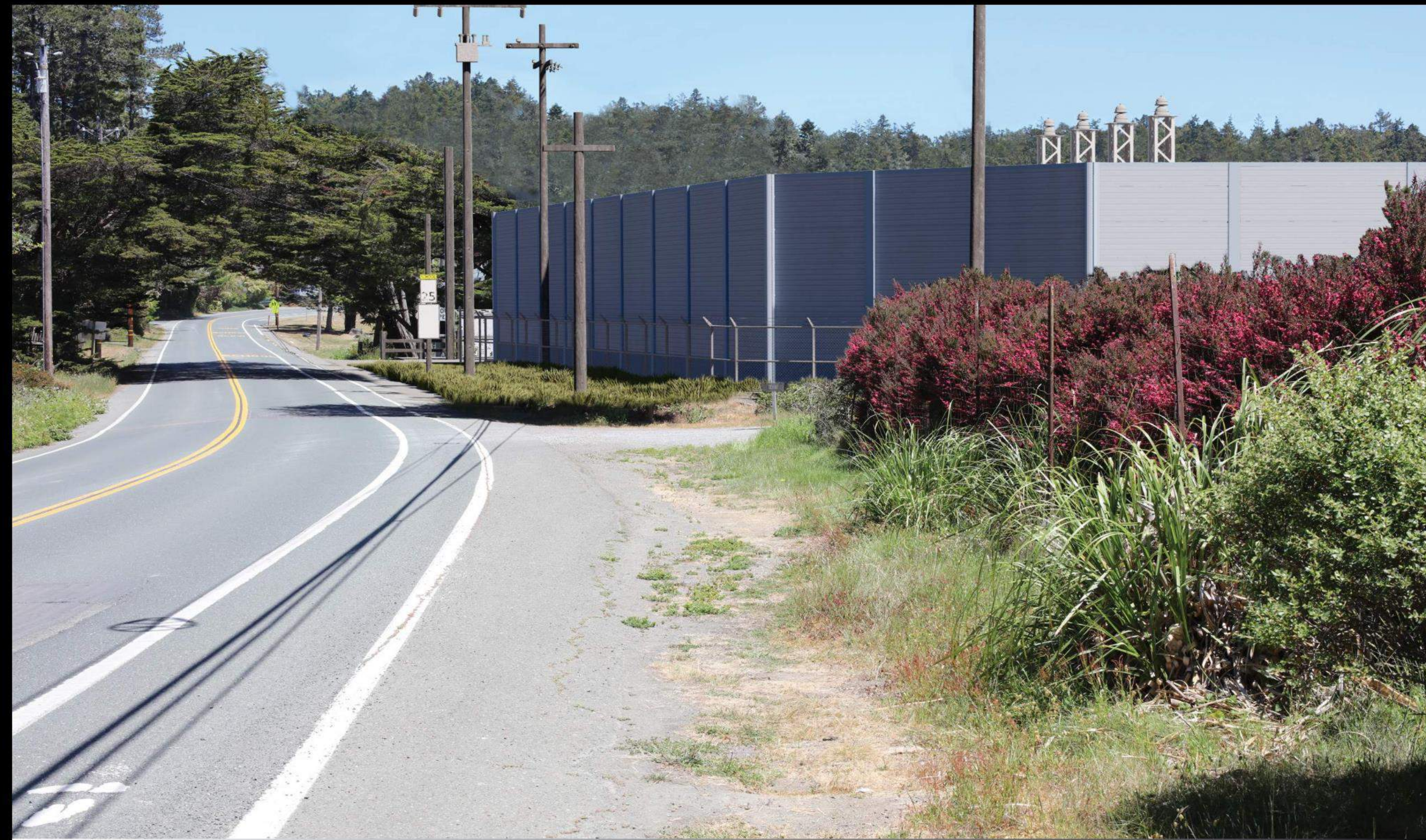
EXISTING WALL / VEGETATION REMOVED
