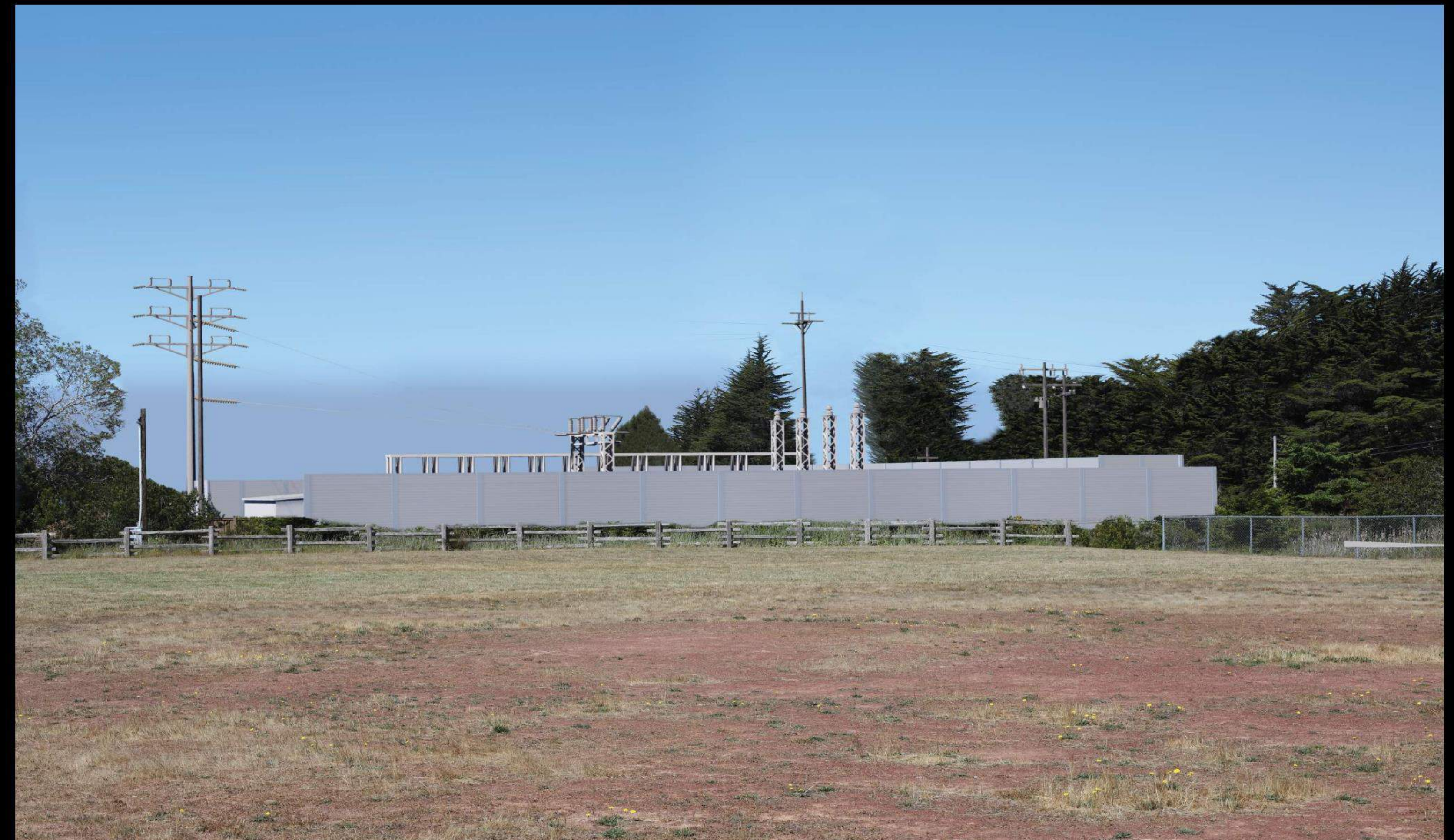
EXISTING WALL / VEGETATION REMOVED
