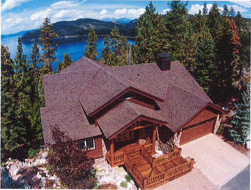
Asphalt Shingle Oakwood Color (Paramount Advantage UL790 Class-A Fire Resistance)
