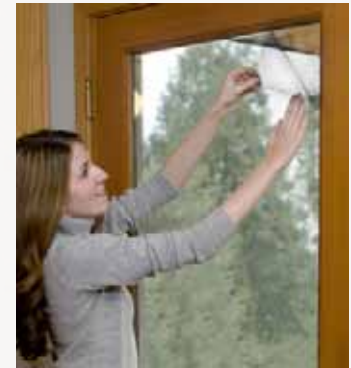
Homeowner installation of low-e interior surface film.
