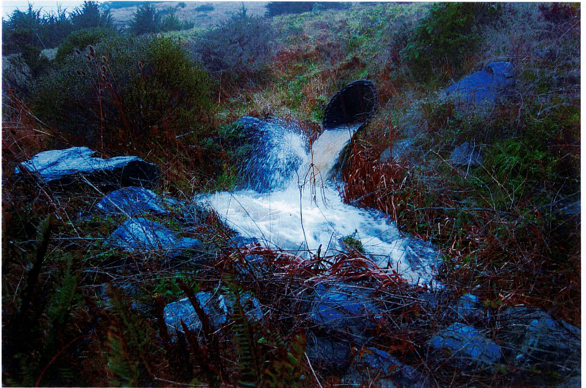
2008 showing the outfall of the diverted storm drain under Highway One, the turn to the south, towards the creek and unpermitted rocks that served to direct the flow.
