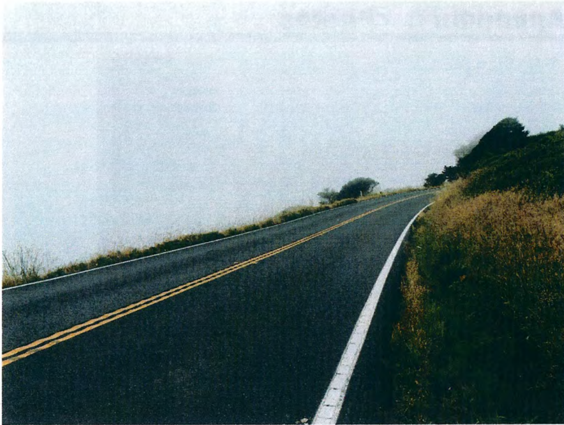
Photo 2. Roadside ditch, D-2, between PM 42.11 and PM 42.26. Photo taken June 13, 2019.
