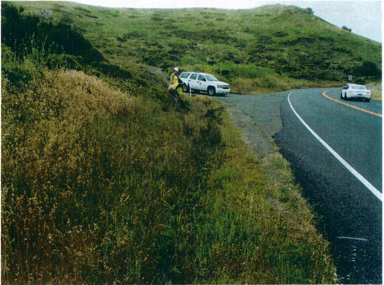
Photo 5. Wetland ditch near PM 41.84 (W-3). Photo taken on June 1, 2017.
