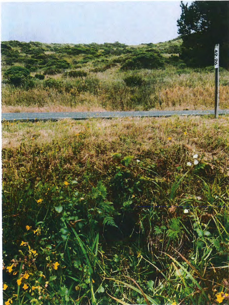
Photo 1. Culvert outlet at PM 42.26 shows OW-4. Photo taken June 13, 2019.
