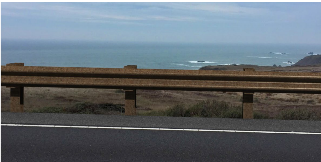
Figure 8 After MGS Installation without staining.
