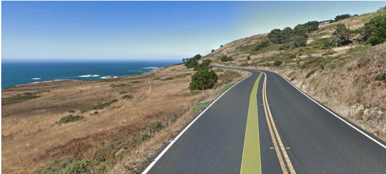
Figure 3. View from SR 1 looking northbound.
