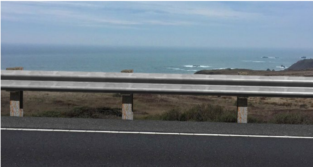
Figure 7 After MGS installation without staining.
