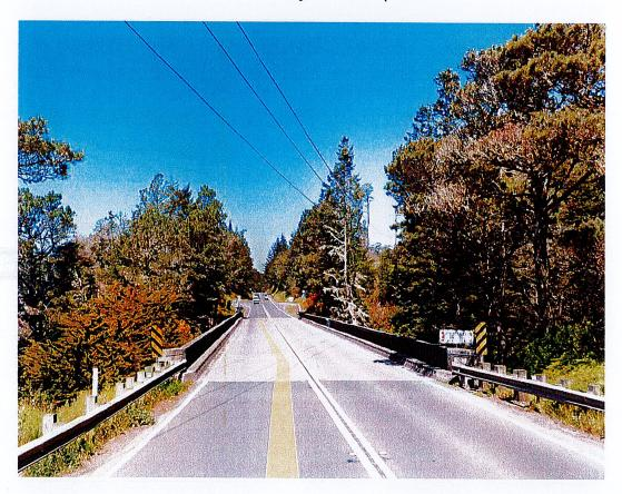
An overhead PG&E powerline will either need to be temporarily raised to a minimum of 100 feet above the bridge deck to provide adequate clearance for the contractor, temporarily or permanently relocated west of the highway or placed underground within the project limits along the west side of the highway. Approximately 28 trees would need to be removed west of the highway to temporarily or permanently relocate power lines west of highway.
