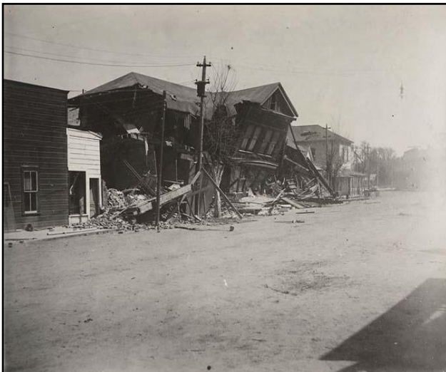
Collapsed building in Willits, after the Great 1906 San Francisco Earthquake.
