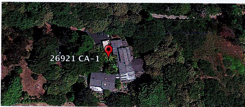
Google Earth image showing the proximity of vegetation to the structures.
