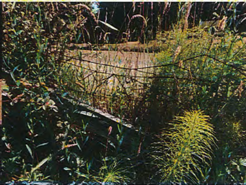
View of existing fence with remnant vegetation
