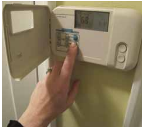
Recommended: [59] Installing a programmable thermostat can help existing systems to operate more efficiently.
