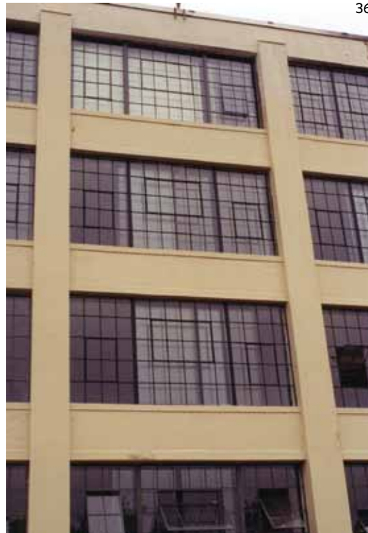
Recommended: [36-38] Original metal windows were retained and made operable during the rehabilitation of this historic mill complex. Installing patio slider doors as interior storm windows was a creative and successful solution to improve the energy efficiency of the existing windows.
