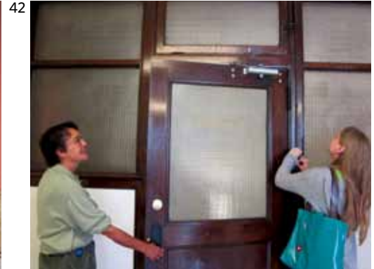
Recommended: [43] The wall and door glazing ensures that the corridor receives natural daylight and the operable transom helps air to circulate in this historic office building.
