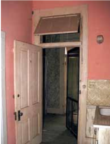
Recommended: [42] Transoms and screen doors are distinctive and practical features that provided cross ventilation in this historic hotel.
