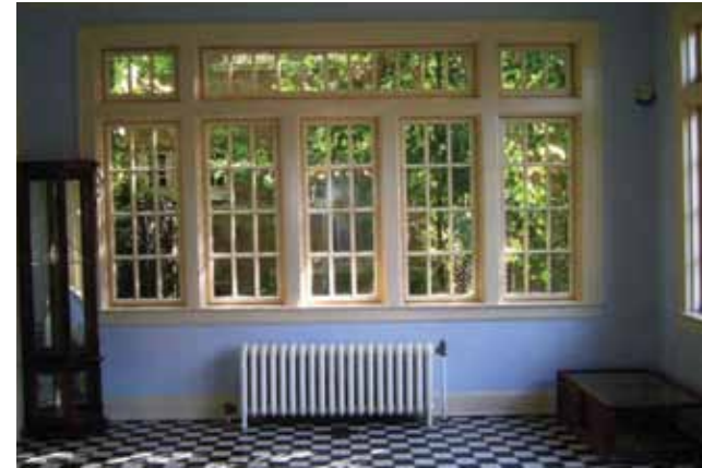
Recommended: [60] Original radiators that are still functional and efficient were retained in the rehabilitation of this historic house.
