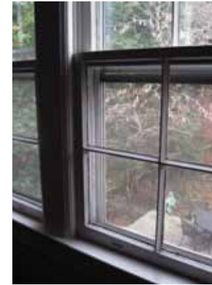
Not Recommended: [31-32] Ill-fitting exterior aluminum storm windows viewed from both inside and outside are clearly not energy efficient.
