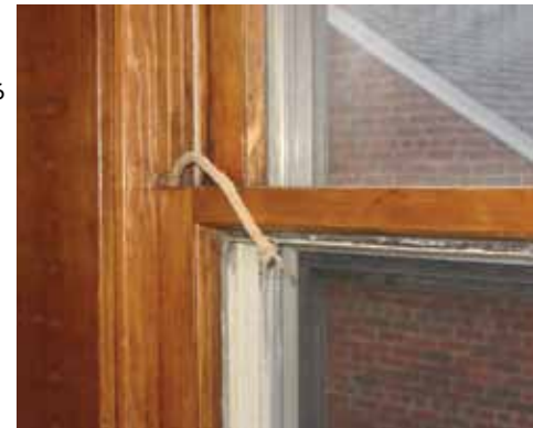
Not Recommended: [27] A broken sash cord can be repaired easily and does not justify replacement of the window.
