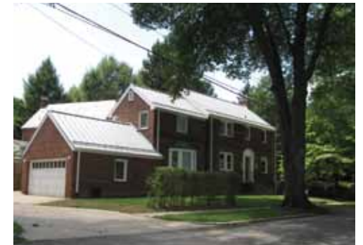
Not Recommended: [88] This new, cool white metal roof is not an appropriate material or color for this historic mid-20th century house.
