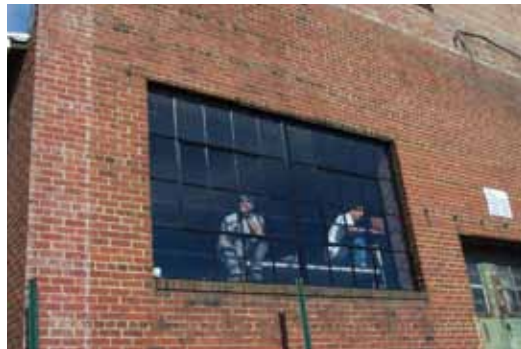
Recommended: [33-35] Original metal windows were appropriately repaired as part of the rehabilitation of this historic industrial building.
