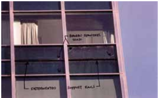
39 Recommended: [39-40] The original windows, which were deteriorated beyond repair, featured a dark tint. They were replaced with a slightly lighter-tinted glazing to improve daylighting in this mid-century modern office building.
