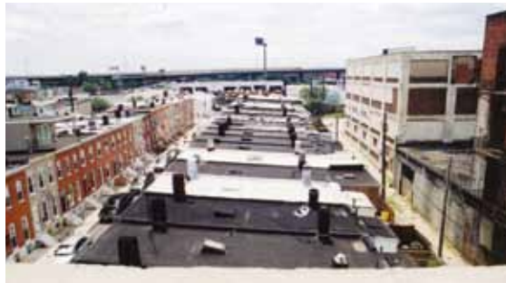
Recommended: [85-86] A cool or green roof is best installed on a flat roof where it cannot be seen from the public right of way and will not negatively impact the character of the historic building.
