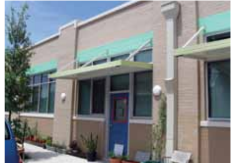
Recommended: [107] Traditional canopies compatible with the industrial character of this former factory building were installed when it was converted for residential use.
