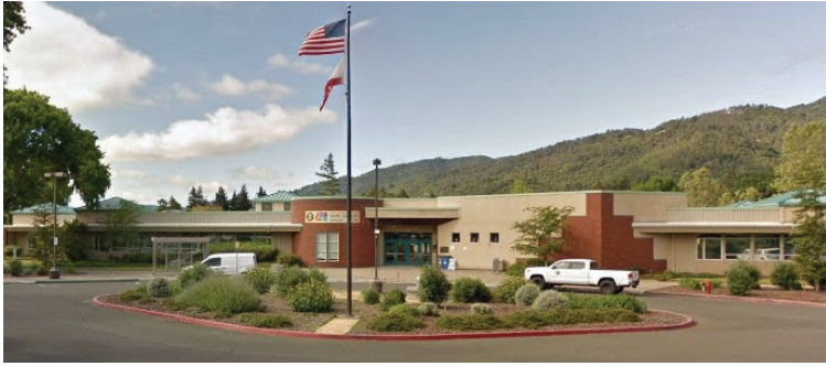
Mendocino County Administration Center, Ukiah
