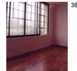
Recommended: [36-38] Original metal windows were retained and made operable during the rehabilitation of this historic mill complex. Installing patio slider doors as interior storm windows was a creative and successful solution to improve the energy efficiency of the existing windows.
