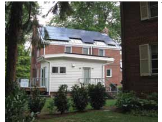
Not Recommended: [75] Solar roof panels have been installed at the rear, but because the house is situated on a corner, they are highly visible and negatively impact the character of the historic property.
