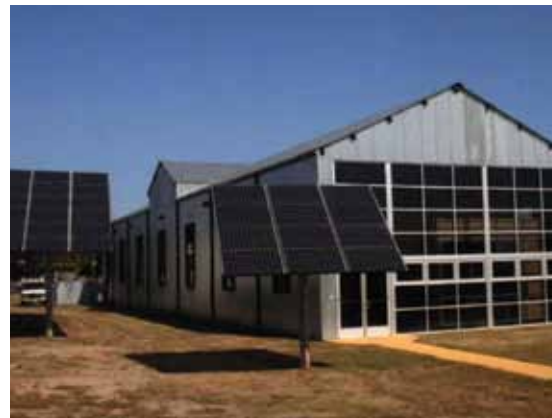
Recommended: [74] Free-standing solar panels have been installed here that are visible but appropriately located at the rear of the property and compatible with the character of this industrial site.
