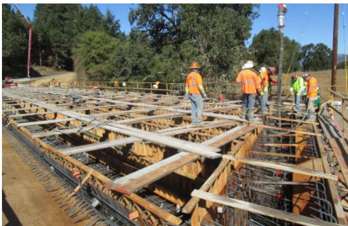
Department of Transportation Bridge Crew during Davis Creek Bridge construction project.
