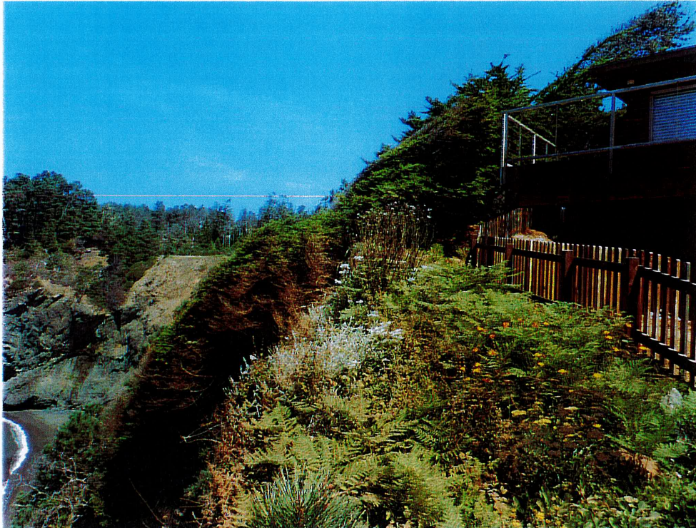
Figure 6. Looking north past the northwest corner of the residence. Native vegetation can be seen directly adjacent to the northern side of the residence. Leafless branches of the fir trees at the lower middle of the photo show where vegetation is absent due to the landslide.
