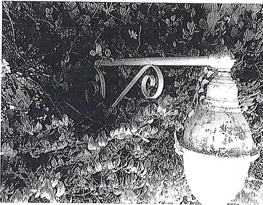
Figure 9 Old Mendocino teardrop streetlight and decorative cross arm used before the cobra-head streetlights of the 1960s
