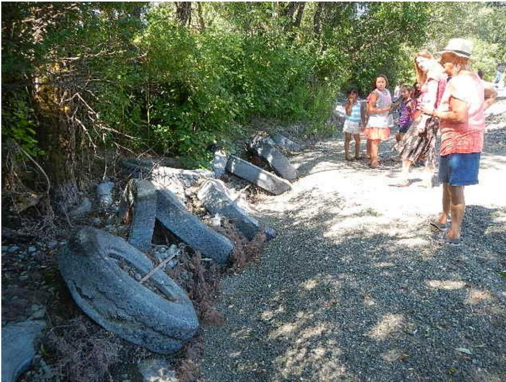
**Figure 4. Truck tires cabled together to stabilize the banks of Town Creek. June 7, 2016.**
